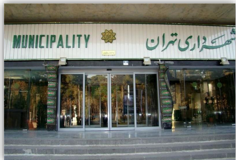
Tehran Municipality Building - Tehran
